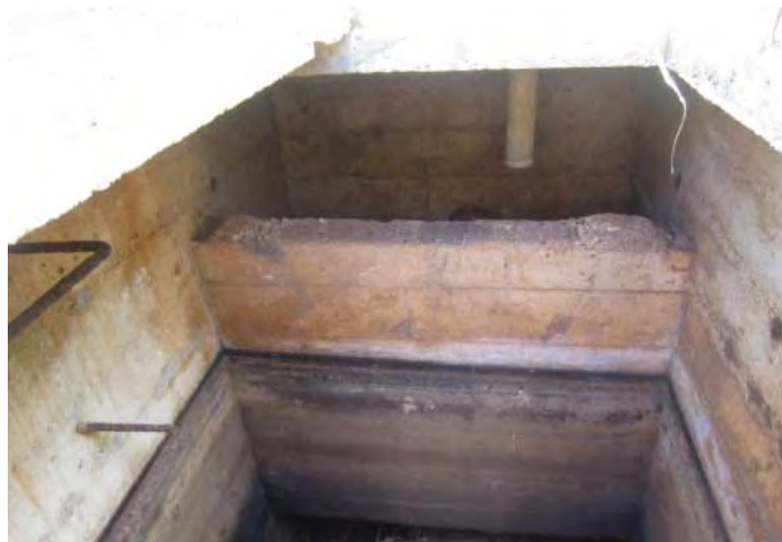
Figure 5.363. Feature VI-33, septic tank interior (2011).
