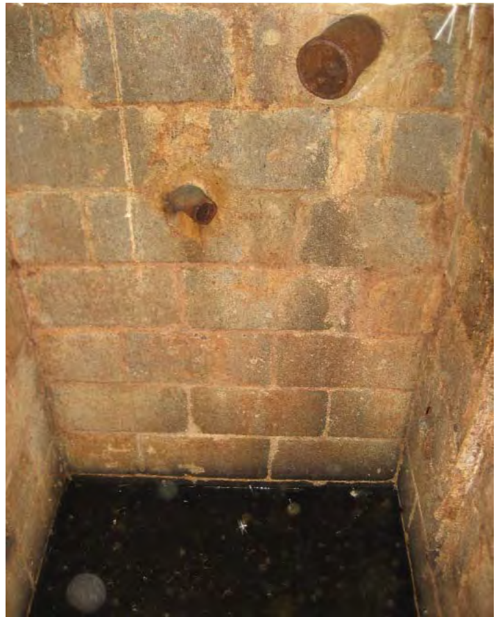
Figure 5.108. Feature III-5, septic tank interior (2009).
