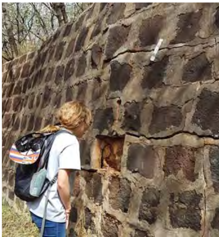
Figure 6.20. Spalling rock wall (Feature V-15) in 2017.
