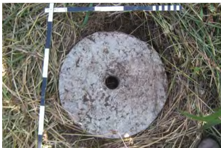
Figure 5.76. Feature II-21, concrete post support (2011).
