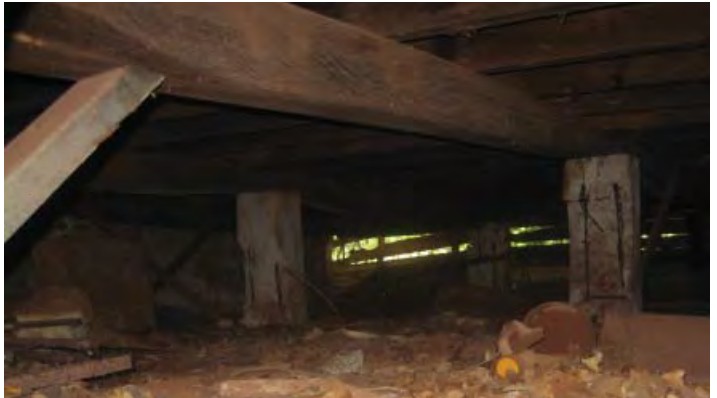
Figure 5.261. Feature VI-1, concrete footers and wood posts(2008).
