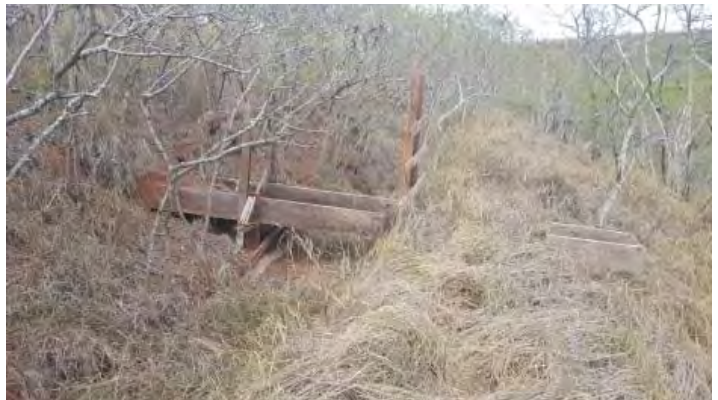
Figure 5.542. Feature L-1f, wood flume crossing ditch (2017).
