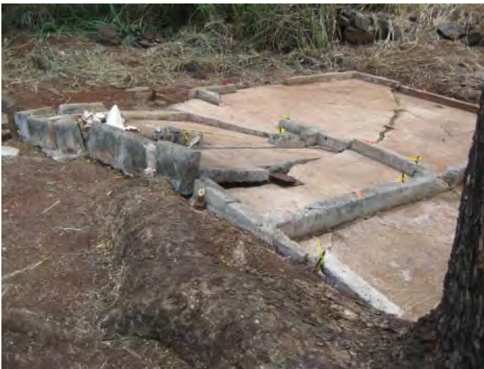
Figure 5.345. Feature VI-32, latrine and shower building foundation showing damage from tree roots (2011).
