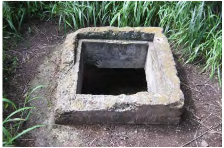
Figure 5.478. Feature VII-3, detail of septic tank opening (2008).
