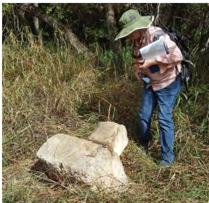
Figure 5.334. Feature VI-29, displaced concrete footer (2017).
