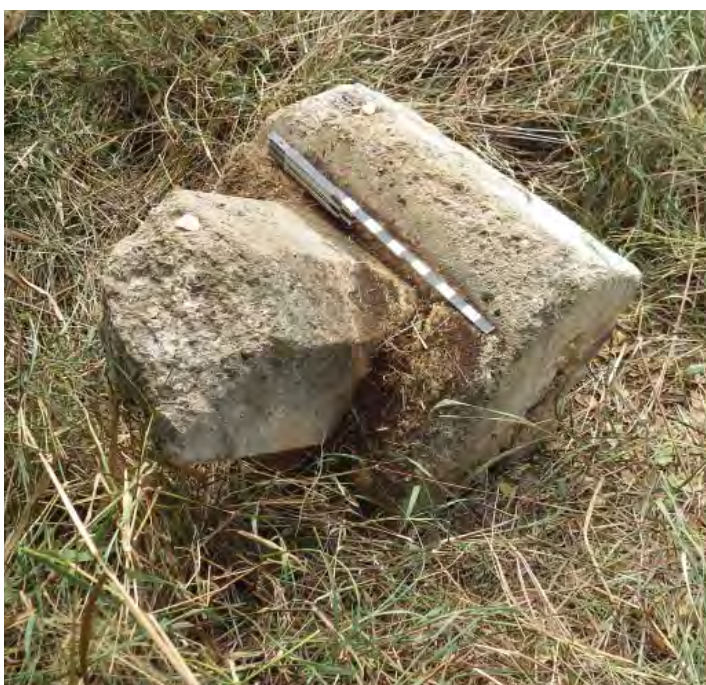
Figure 5.333. Feature VI-29, displaced concrete footer (2017).
