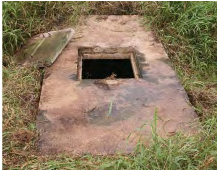
Figure 5.106. Feature III-5, septic tank (2009).
