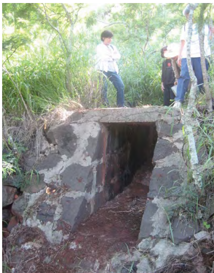
Figure 5.537. Feature L-1d, ditch outlet gate (2008).
