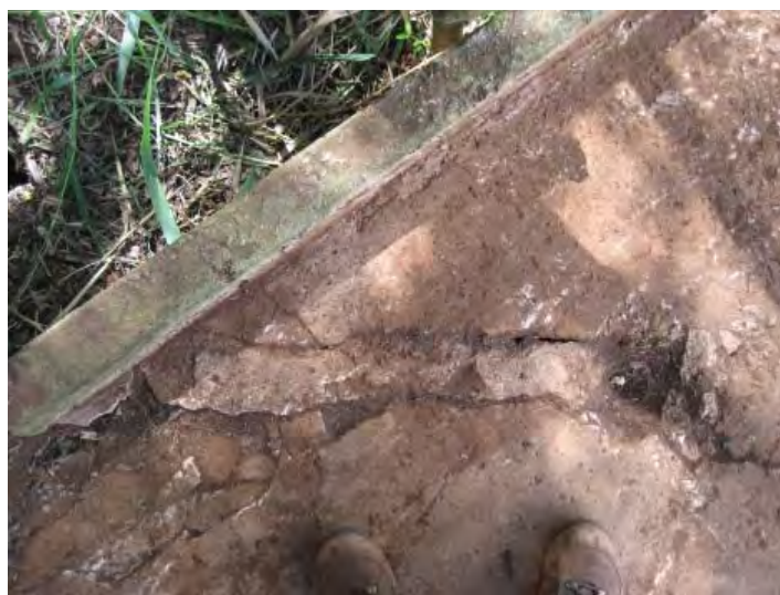
Figure 5.156. Feature V-1, concrete patch in west extension slab (2009).
