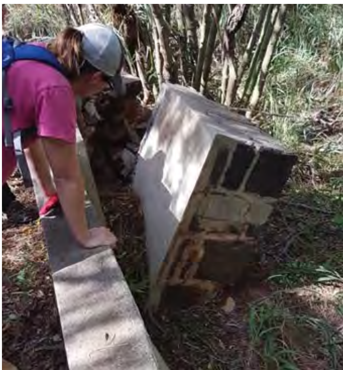
Figure 6.19. Tilted pier of the aqueduct (Feature L-1b) in 2017.
