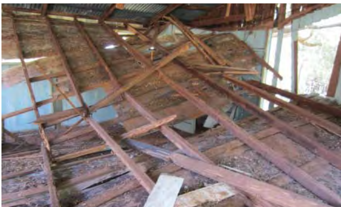
Figure 5.603. Feature M-6, collapsed ceiling of standing building on concrete foundation of Feature VI-1 at chicken farm (2012).
