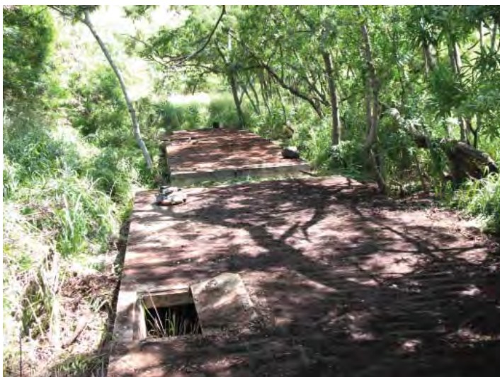
Figure 5.473. Features VII-1 and VII-2, septic tanks (2008).
