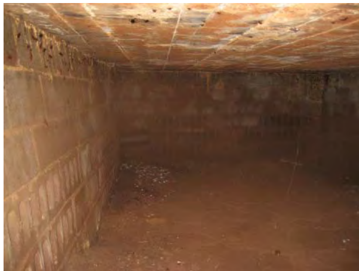
Figure 5.367. Feature VI-34, septic tank interior (2008).
