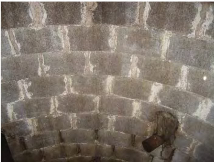
Figure 5.94. Feature III-3, cesspool interior (2014).
