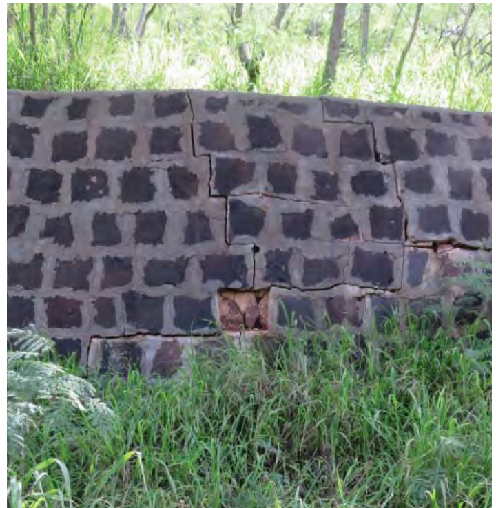
Figure 5.198. Feature V-15, missing veneer rock and cracks in rock wall (2014).
