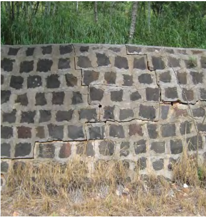
Figure 5.197. Feature V-15, cracks in rock wall (2008).
