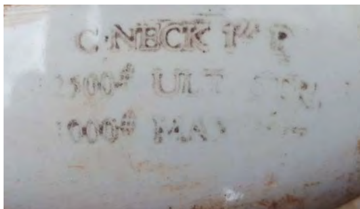
Figure 5.506. Feature VII-16, detail of ceramic power pole insulator (2017).
