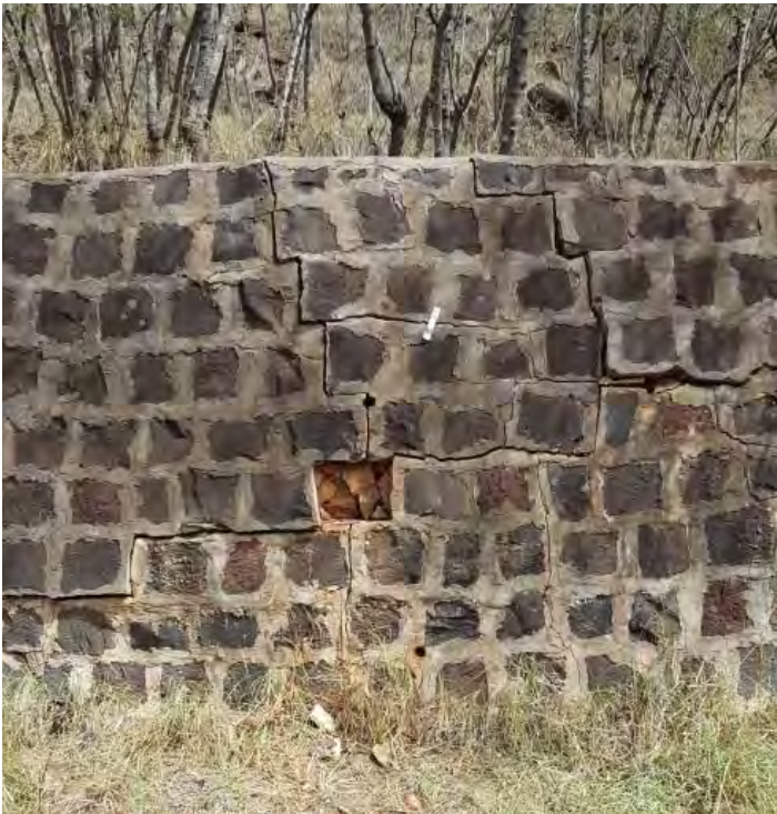
Figure 5.199. Feature V-15, missing veneer rock and cracks in rock wall (2017).
